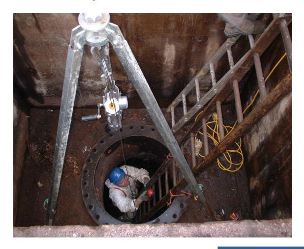
Planned shutdown works incorporating power outage at the North Wall Generating Station in Dublin provided an opportunity to inspect the cooling water culverts. ESB engineers carried out a visual internal inspection of the reinforced culverts and discovered that two joints had failed were allowing water to seep from the structure.
