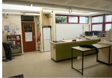
Larsen Contracts have completed a third anti-slip safety floor for Skerries Community College. Previously the PVC sheet vinyl in the metalwork and woodwork rooms had become a trip hazard due to be-bonding. Larsen proposed a MMA fast curing, anti-slip, decorative Quartz screed. Works to both rooms were completed in one week during the school holidays.
