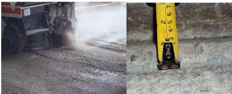
Concrete Repair /Post Scabbling
