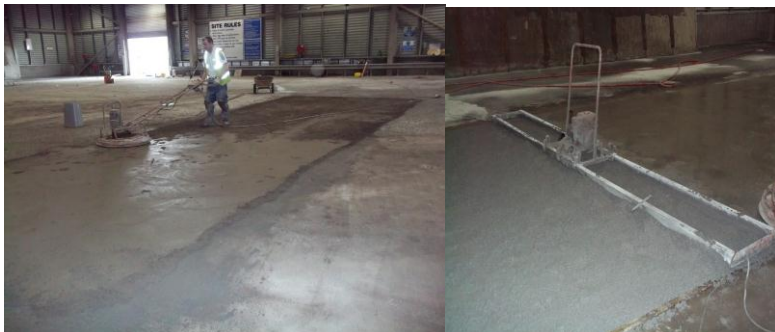
Application of Densitop to Concrete flooring at Dargan Road
